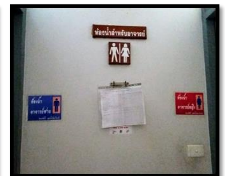
Figure 9: Rest Rooms (Khelang Campus)
